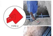
Patented Type 1 and Type 2 non-metallic **STA-DOWN™ CRD** can be used with all manufactured chairs, spacers, racks or grids. Both CRD's are made entirely of injection-molded polypropylene plastic making underground electrical conduit installations safer, easier and more economical. **STA-DOWN™ CRD**'s unique designs are easily inserted into the ends of 1-1/2" schedule 40 PVC conduit, saving an average of 25-28% less labor in the field.
