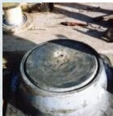
Hammer cushion set in pile cap.
