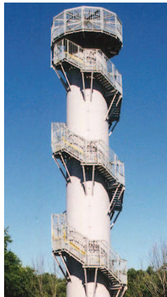
A system of FRP spiral stairs and landings supported by EXTREN® beams circle the Cordova Park Observation Tower at Red Rock Lake near Des Moines, Iowa.
