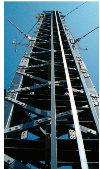
A 62' (19.5m) tall weather tower at Vandenberg Air Force Base near Santa Barbara, California is composed of EXTREN® structural shapes, ladders and DURADEK® pultruded grating.
