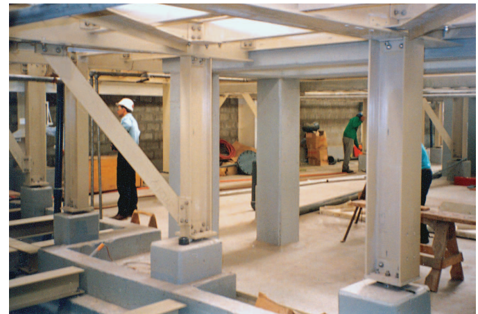
EXTREN® structural shapes were used in a SXEW copper refinery because of the highly corrosive environment.
