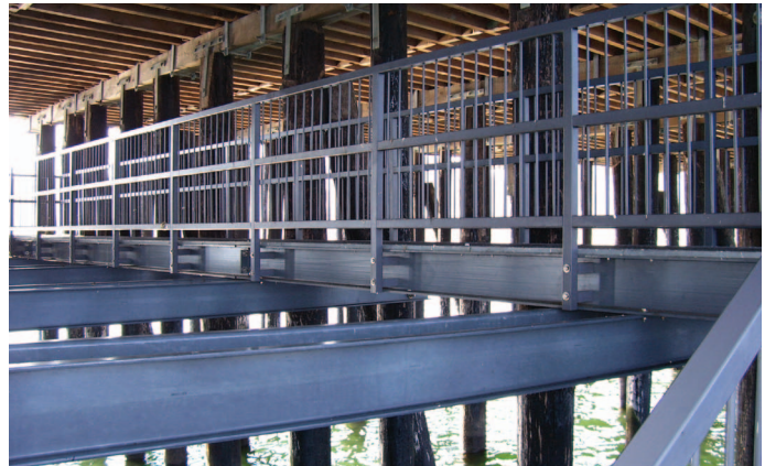
The Avila Beach Pier in California was reconstructed using EXTREN® structural shapes for support, DURADEK® pultruded grating, stair treads and handrail.
